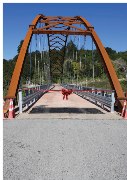
The new permanent Te Reinga Bridge is now officially open.
