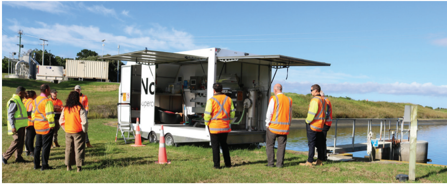
Wairoa District Council elected members and staff visited the ultraviolet filtration trial at the Wairoa wastewater ponds.
