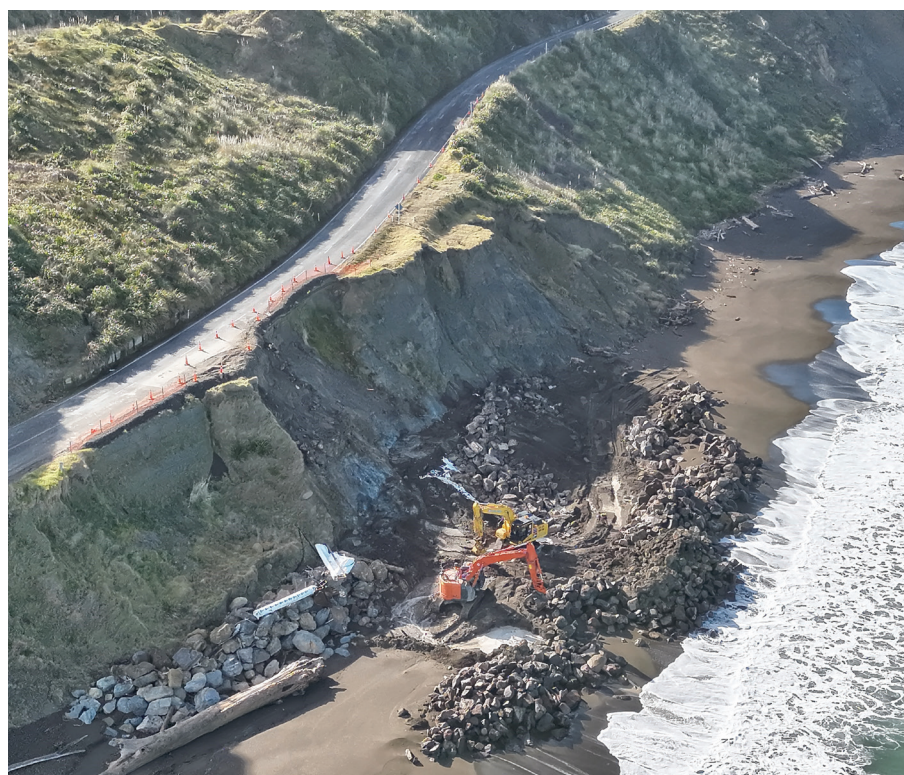
Coastal resilience using rock revetment along Black's Beach, Mahia
