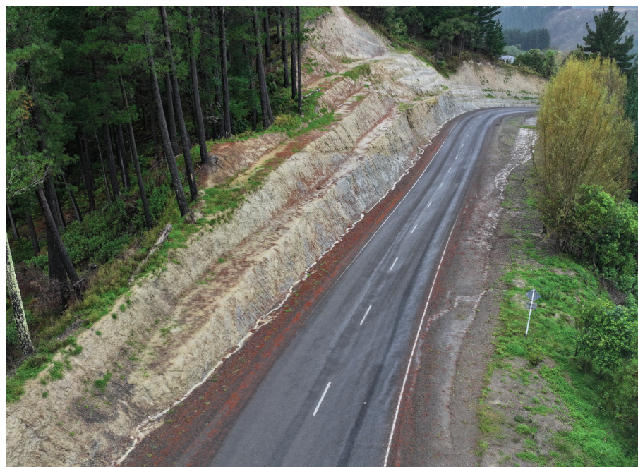
A land slump took out half the corridor on a section of Cricklewood Road, with the road realigned by retreating into the hill.
