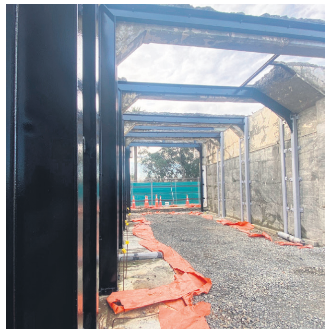
Work on the main street Te Wairoa E Whanake, revitalisation project is set to ramp up this month.
