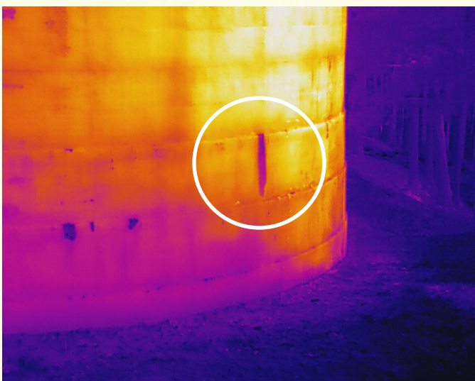
The dark spot on the reservoir marks a water leak, easily picked up by the thermal imaging capability of the drone.
