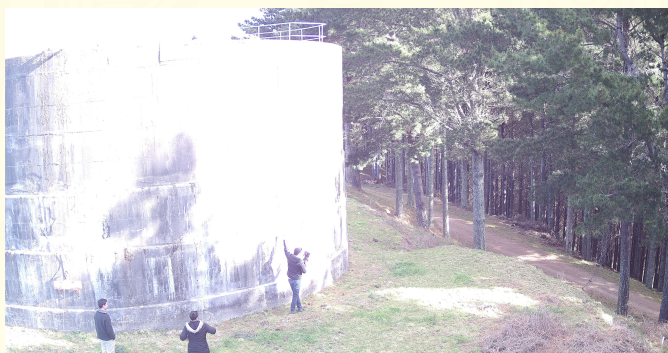
No leakage visible in the image without the thermal imaging ability.
