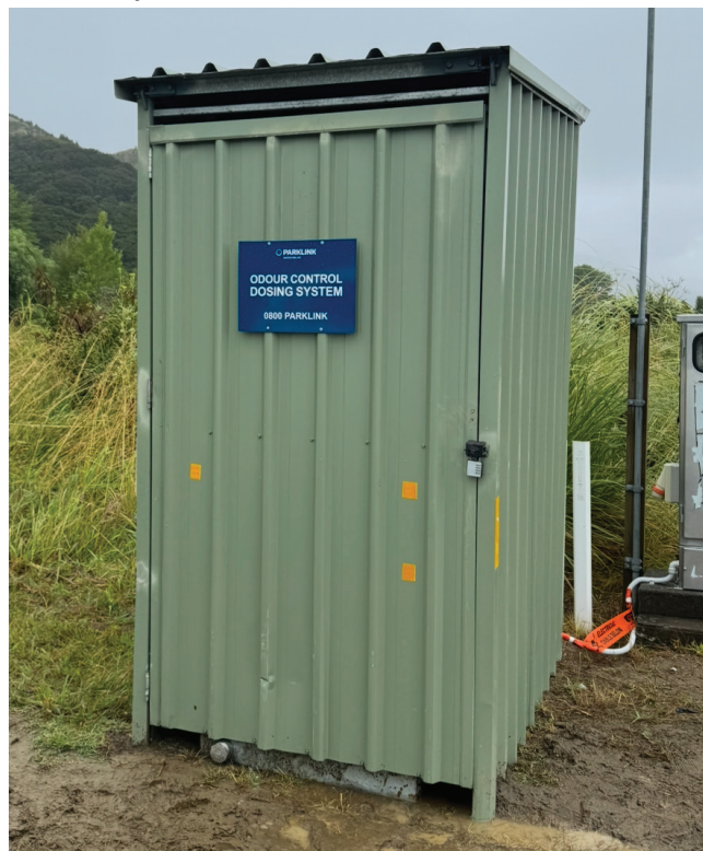
Opoutama – odour control, installed December 2024 – doses magnesium hydroxide to help control odour.
