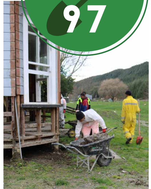
Under house silt removal is a team effort.
