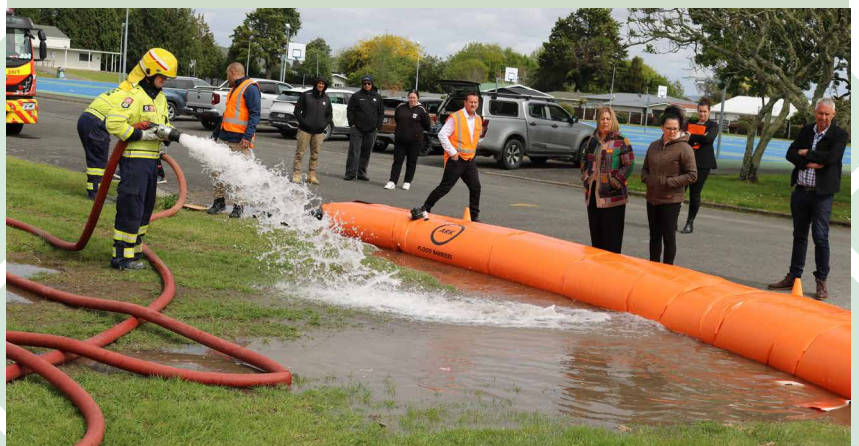
A demonstration of reusable mobile stop banks was held in Wairoa recently.
