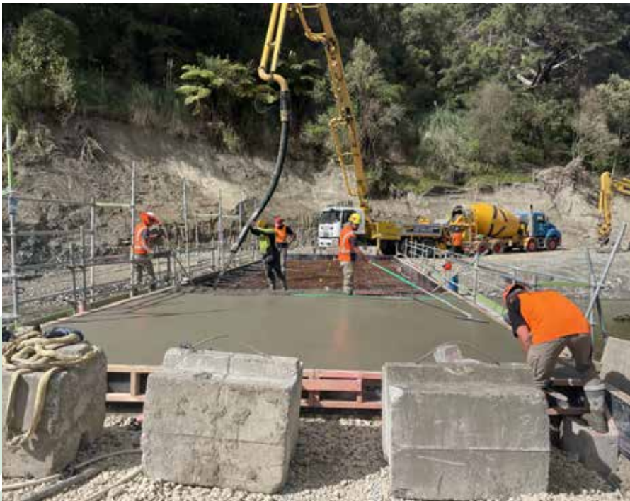
The concrete deck of the Glenbrook river crossing being poured.
