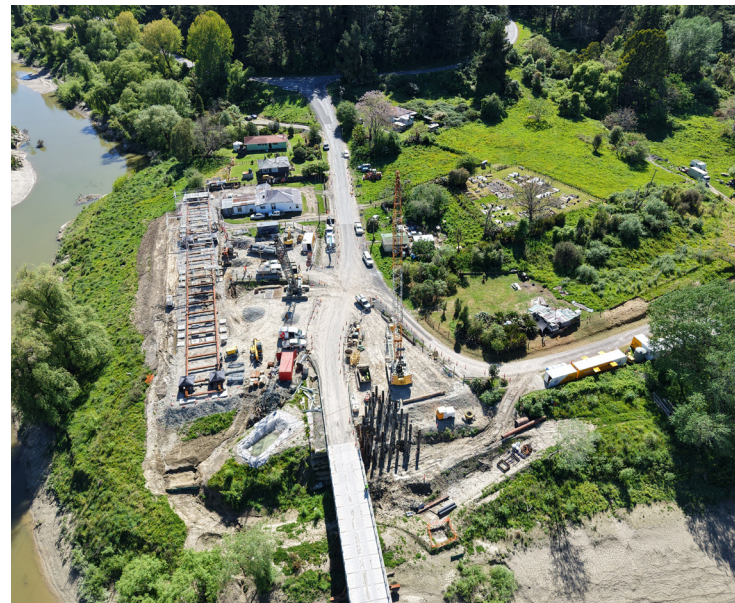
The new permanent Te Reinga Bridge is being built on site, pictured to the left of the photo, with ground improvement piles (to the right of the temporary bridge) completed. Thank you to residents and landowners who have allowed the contractors to use their land for the assembly of the bridge.
