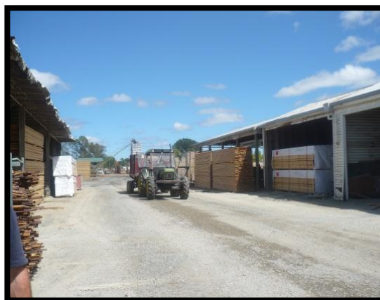
Photograph 6: General building structures at East Coast Lumber
