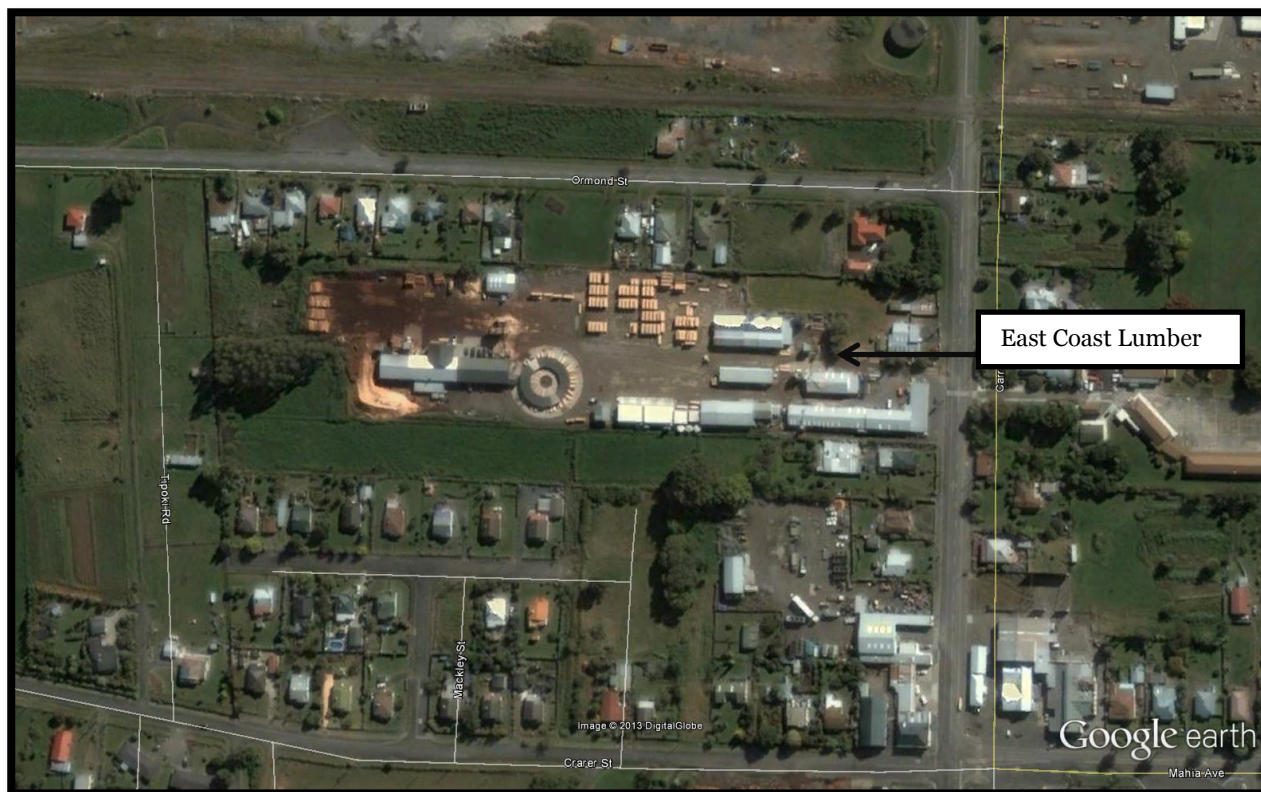
Figure 2: East Coast Lumber Site
